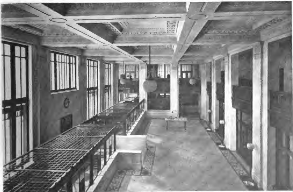
Banking Room from Mezzanine Floor.
